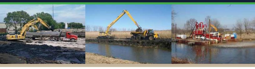
Simultaneously to dredge operations, the Roxana Marsh area was mechanically excavated to a design elevation, and then backfilled using clean sand. Once the excavation and sand placement was completed, all of the areas that were disturbed during the remediation process were restored. This included planting native trees and shrubs to replace the vegetation that was removed during excavation.
